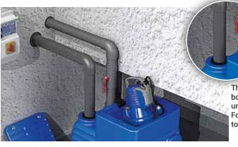
Connect the wastewater intake lines and the breather line (if
