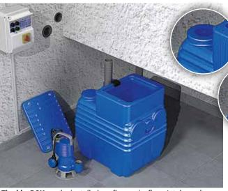
Before putting the pump in place, drill holes in the sides of the tank in the chosen points using a flared grinding tool of the right diameter for the pipe to be used.
